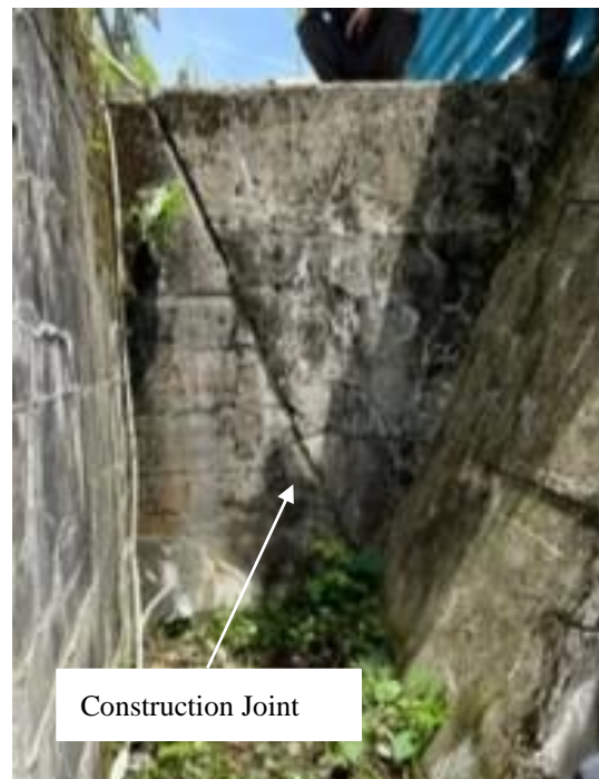
Fig. 2 Target Retaining Wall
