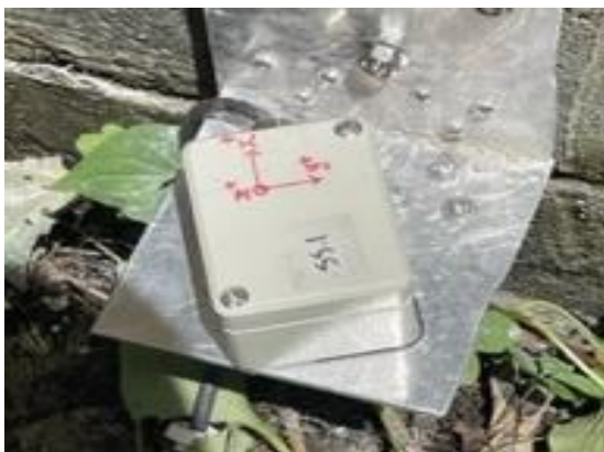
B) Bottom Installation
