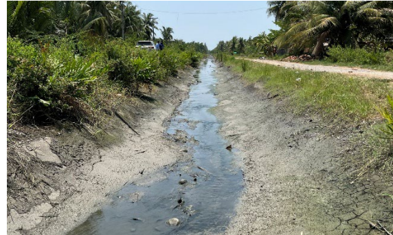
Fig. 1 Drainage canal in Phetchaburi province
