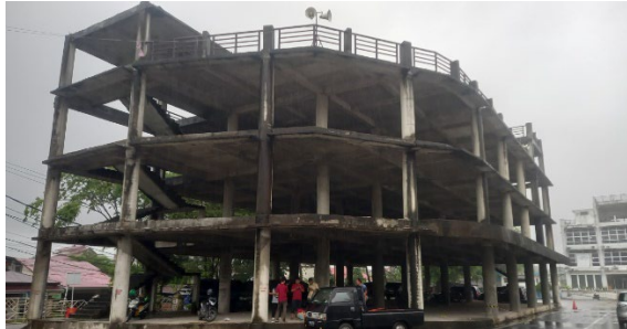
Fig.1 Existing conditions of the BPBD building
