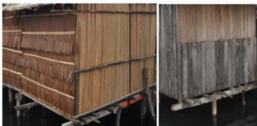
a. Wall material from gaba-gaba (sago palm stem) and timber blade.
