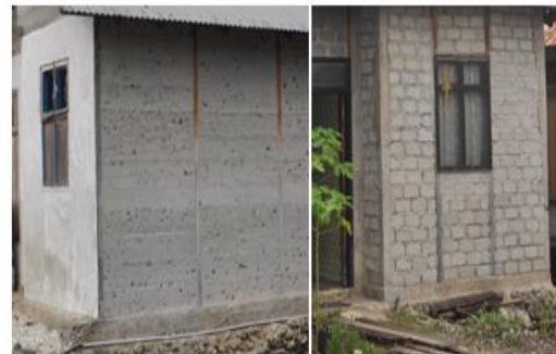
c. Wall material from cast wall and brick.
