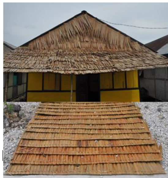
Fig 5. Roof material of Bajo house.
