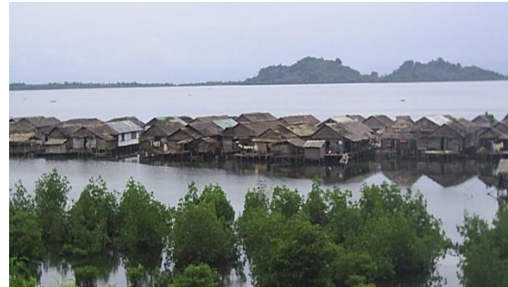
a. The condition of Bajo settlement in 2006.
