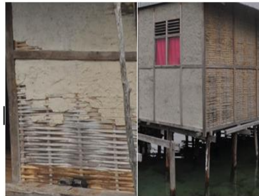
b. Wall material from the woven bamboo blade with plastering.
