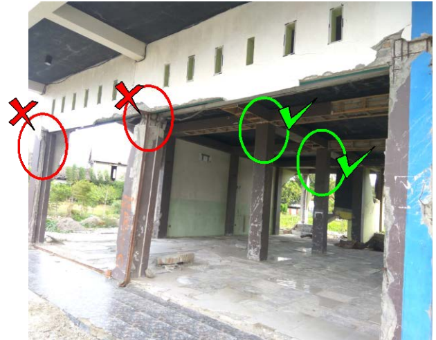
a. Damaged out side column
