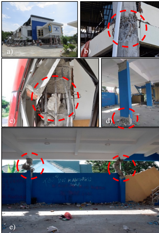
Photo 4 Typical damage of RC structures: a) The first story collapsed due to the soft story, b) Failure of beam-column joint, c) Shear failure of column d) Buckling of longitudinal reinforcements of column e) Shear failure of short columns
