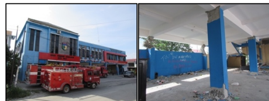
b) The Fire Station building and its damaged columns
