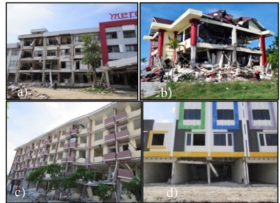
Photo 2 Collapsed and damaged RC buildings: a) Mercure hotel, b) Politic Science Faculty building of Tadulako University, c) Public apartment, d) Shophouse
