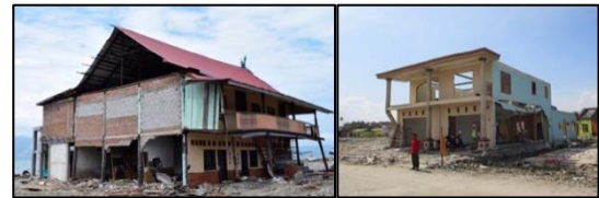
Photo 1 Damage on confined masonry structures
