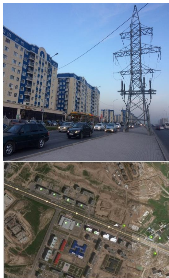
Fig. 1. General view of the 110 kV overhead line power pole installed in the Nursat microdistrict and a geoinformation map based on the danger gradient of electric and magnetic fields
