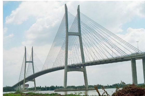
Fig.1 General view of My Thuan Bridge (2000)
