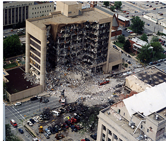
Fig.2 Total collapse of half of the reinforced concrete 9 storey Oklahoma building
