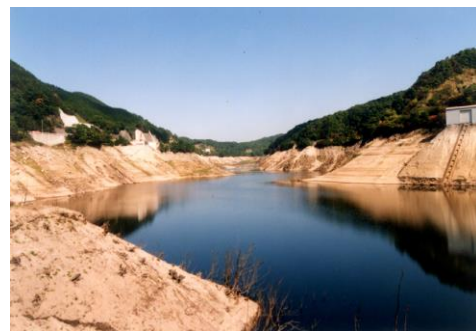
Photo 1 Reservoir slopes exposed when the water level of dam was lowered (reproduced from the River Bureau, Min. of Land, Infrastructure, Trans. and Tourism [14]).
