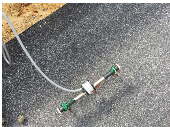
Fig. 2 Detail on installation of string strain gauges
