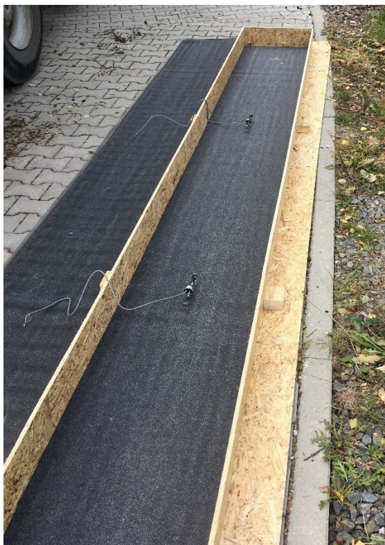
Fig. 1 Installation of string strain gauges
