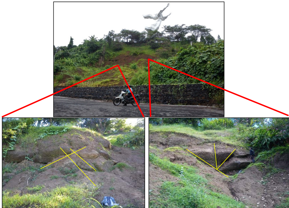
Fig. 2 Discontinuity Condition in Rock Slide Area
