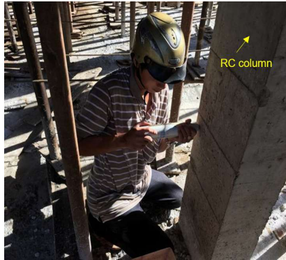
Fig.6 Rebound hammer testing of column
