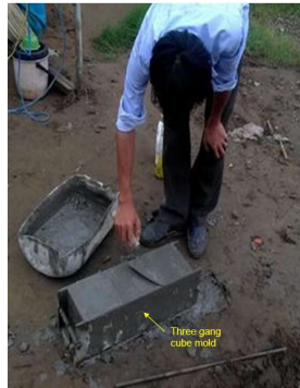
Fig.2 Making on-site concrete specimens
