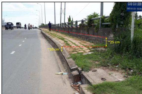
Fig. 2. View of Cai Son Bridge on May 13, 2018 [17]
