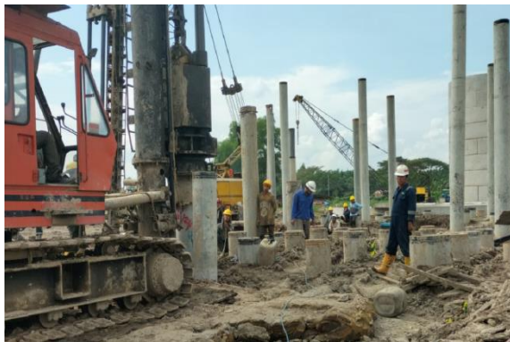
Fig. 1 Multiple Pile Test on Site
