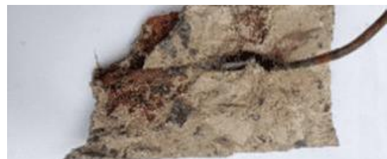
Fig. 16 Beam specimen after breaking
