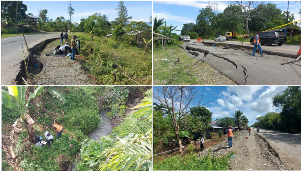
Fig. 5 Landslide condition of study area
