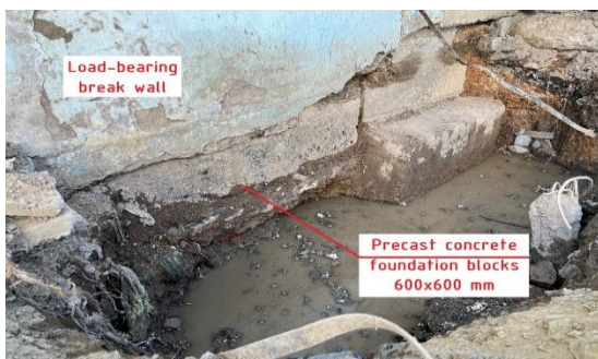
Fig. 3 Test Pit 1 (strip foundation)
