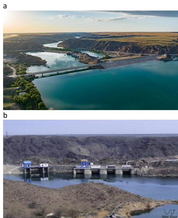
Fig. 1. a) aerial view of the Kapchagay Hydroelectric Power Plant; b) view from the downstream side showing the turbine penstocks and operational spillways.
