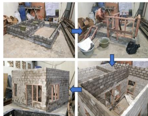
Fig.9 Construction of the brick wall for Specimen OH
