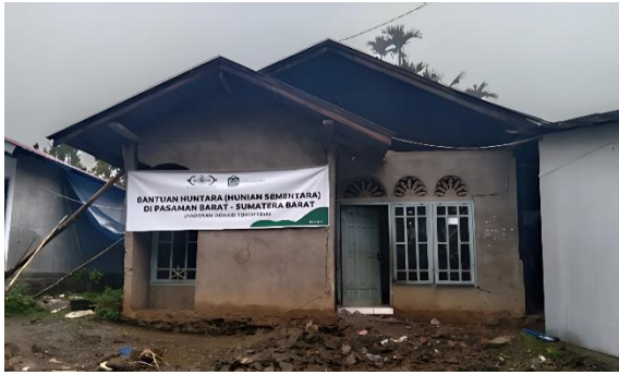
Fig.2 URM hollow brick community house in West Pasaman
