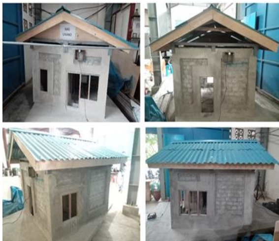
Fig.18 Specimen RH after completion of repair and retrofitting using the ferrocement layers method
