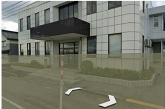
Fig.12 The Three-dimensional inundation hazard map at Street-B where water depth is 1.21m
